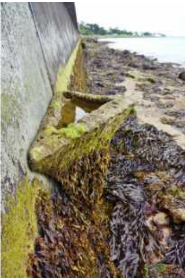
Vertipool in the splash zone - attached to a sea wall. © Artecology
